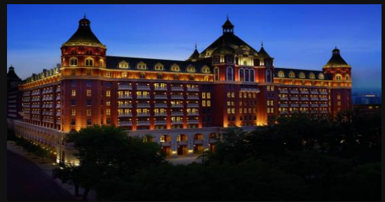
Tianjin Ritz-Carlton Hotel
