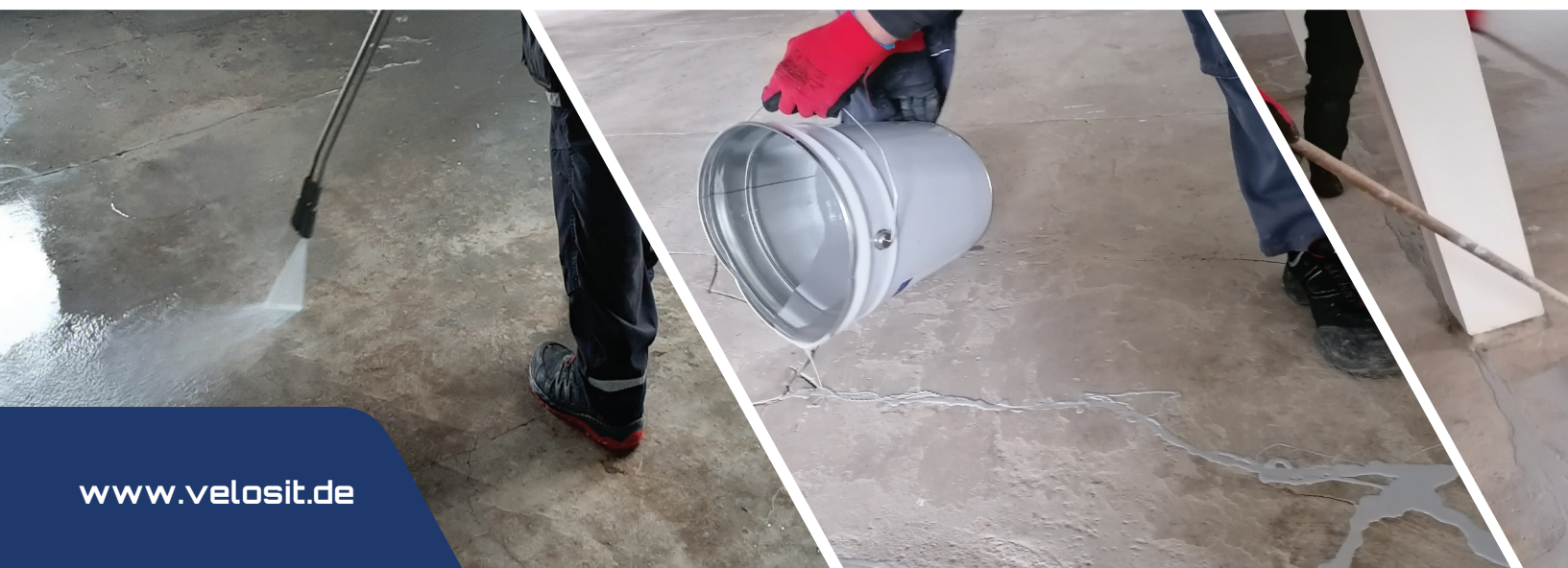
Fig. 1. Cleaning with a high-pressure cleaner.
