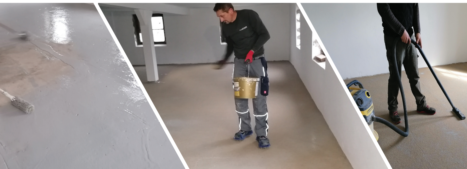
Fig. 4. Full-coverage sanding with suitable quartz sand 0.7 – 1.25 mm into the fresh coating.
